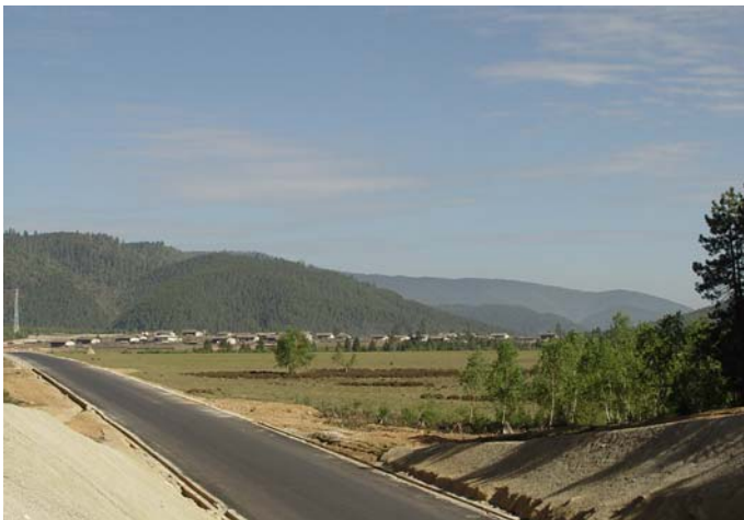
Fig. 2 Looking north to upper Jisha along the new highway, which was cut through the cemetery forest. This road has granted easy access to large areas of pine forest to the south
